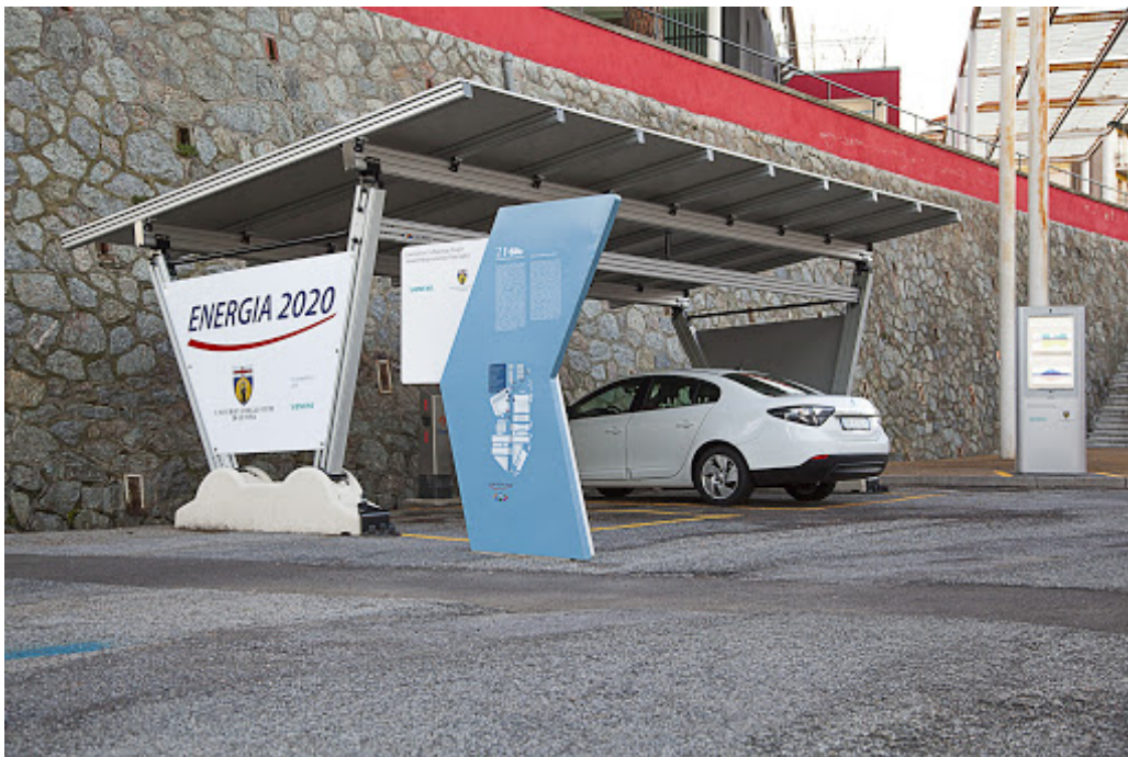
Figure 2.3: The parking lot for e-vehicles.
