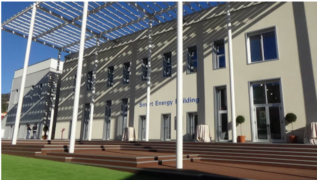
Figure 2.2: The zero-emission building (front view).
